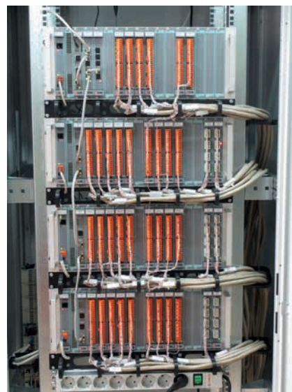
Centralized system example
